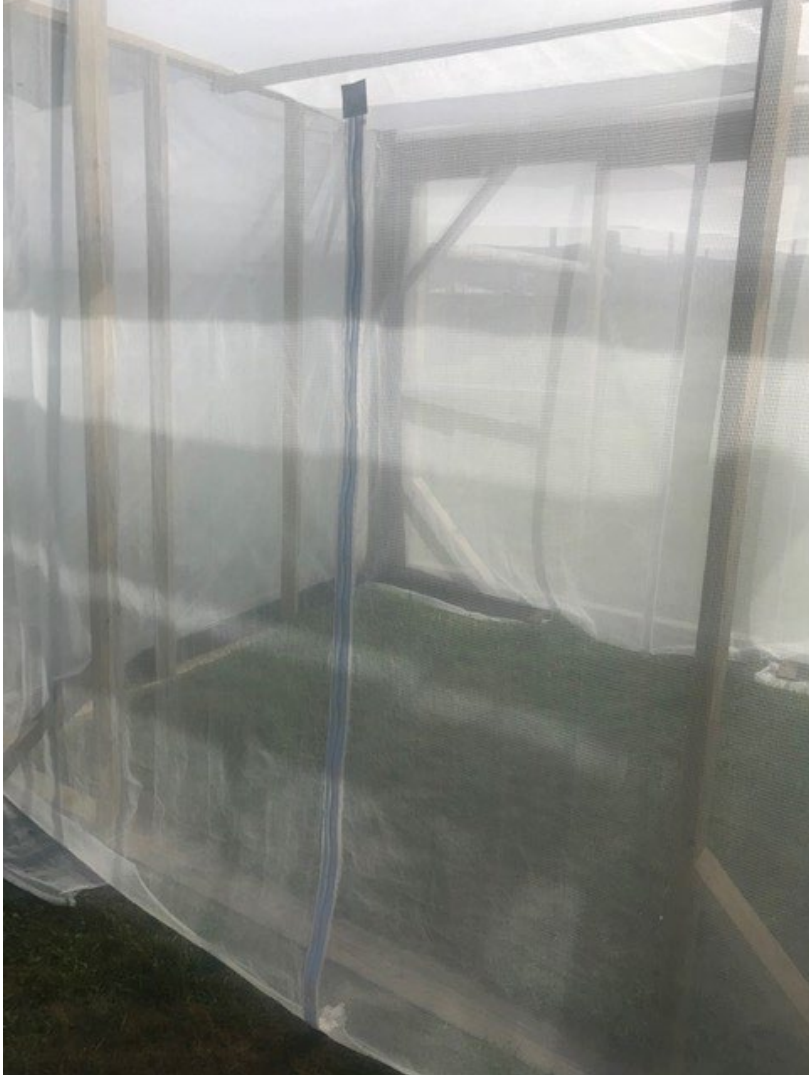
Constructed 10' x 10' Double Entrance
