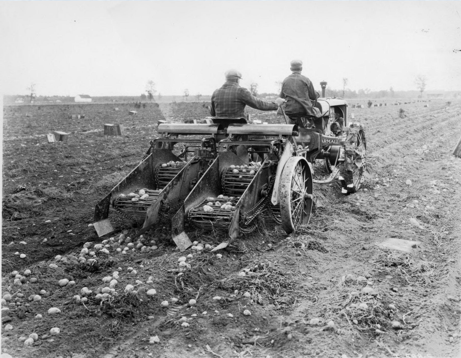
Digger: Dig out and put on surface
